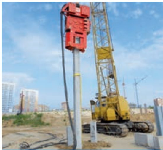
30HV Vibrodriver equipped with Multigrip clamp driving 350 mm square concrete piles in Russia.
